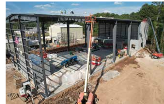
RTI transforms early-stage energy research into scalable, market-ready technologies.
